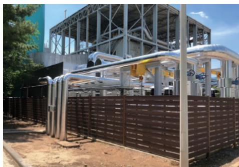
Low-temperature heat recovery from fuel cells in Bucheon
